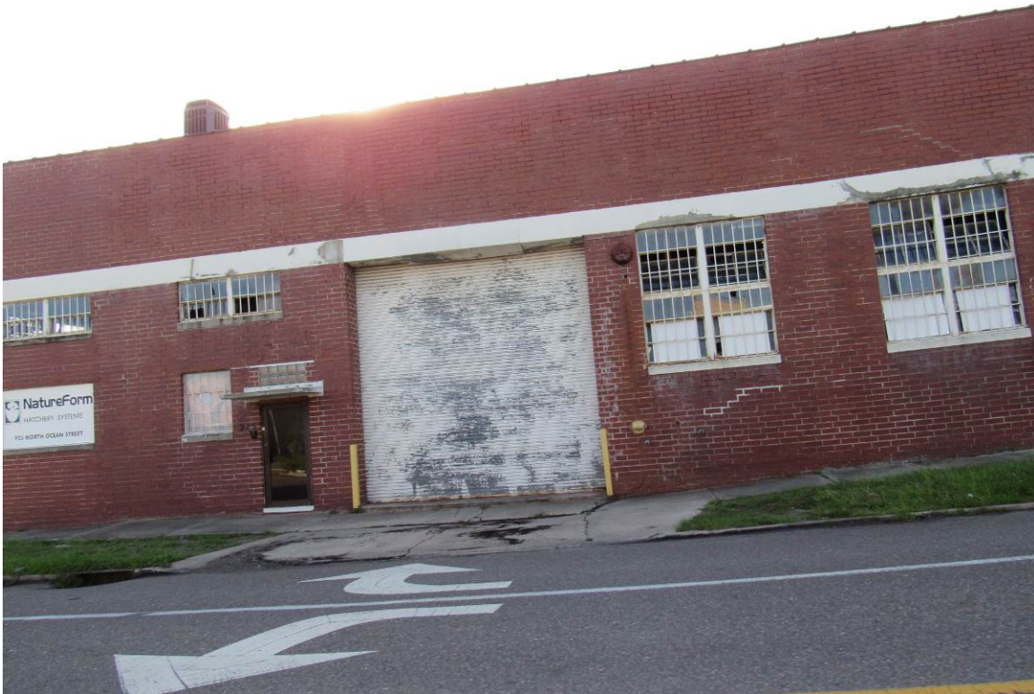
Adjacent commercial building.
