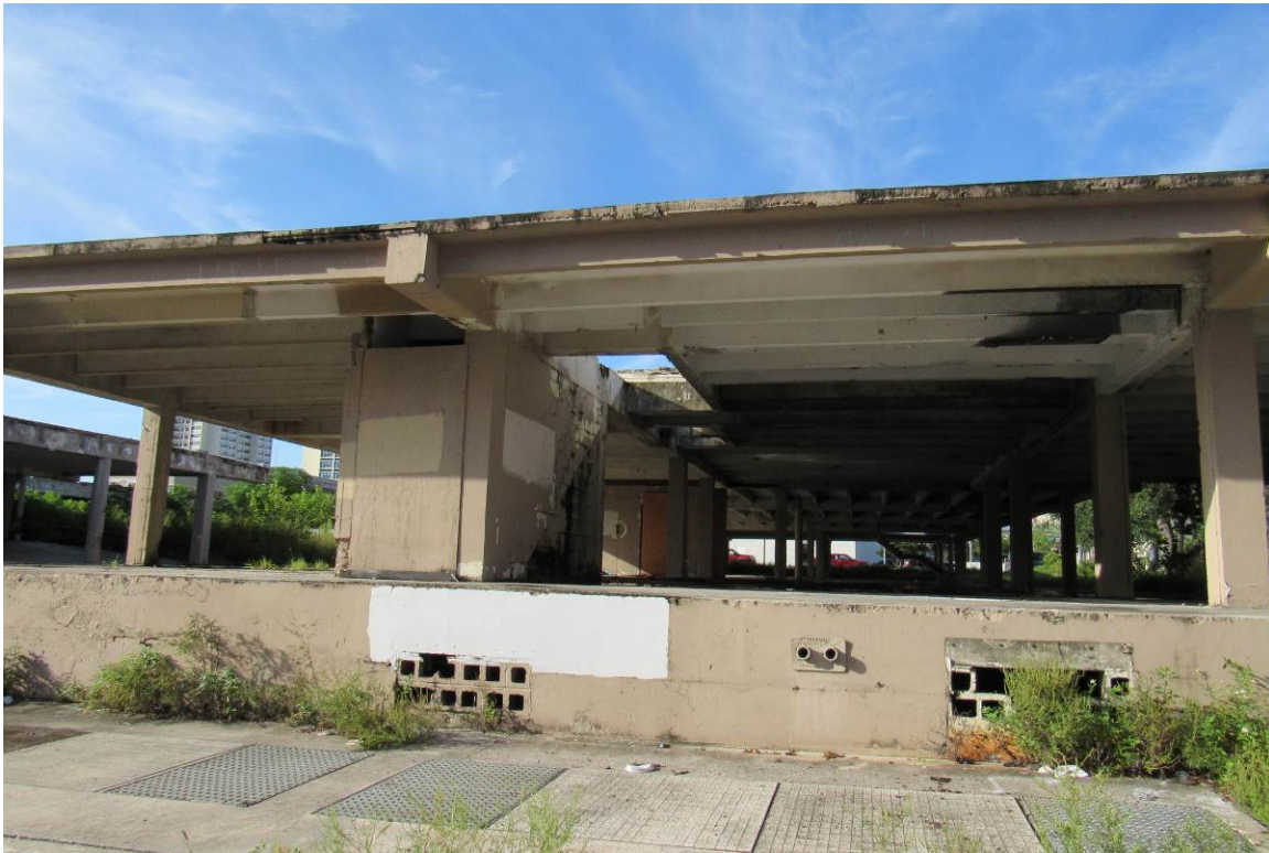
View of existing structure.
