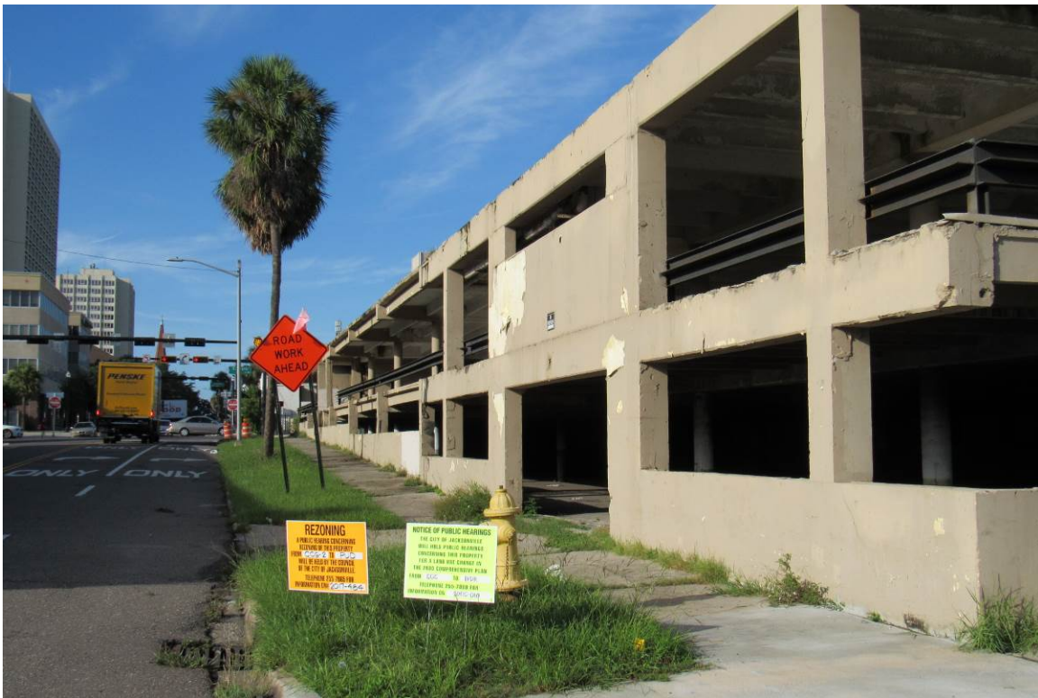
View of existing structure.
